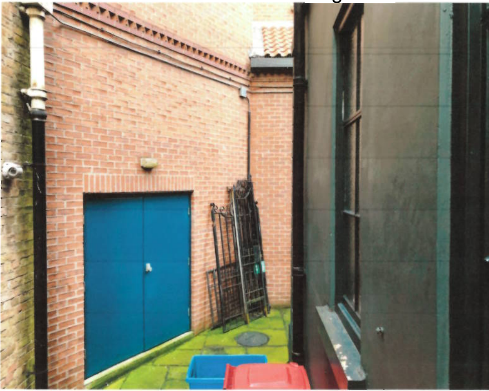
A photograph showing the proximity of the proposed bar and emergency access door to Judges Court's side windows
